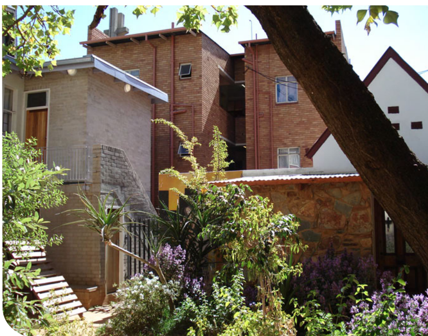
Social housing in Pretoria city centre area
