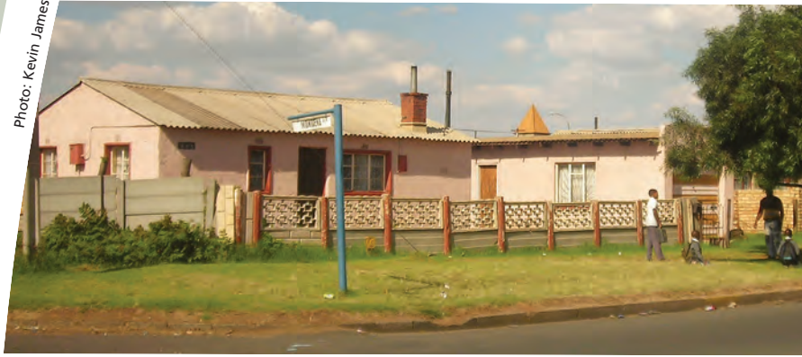
Wattville is an older, established area
