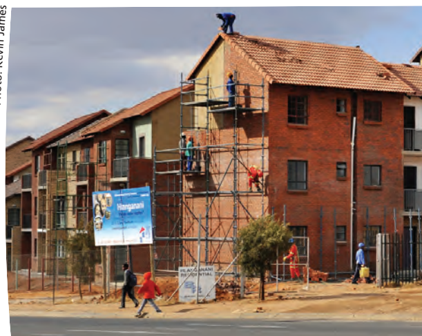
Construction at Cosmo City
