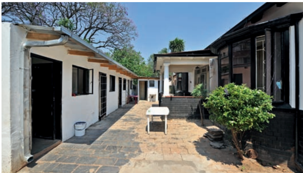
Rows of rooms to rent on the left with shared ablutions at the end.
