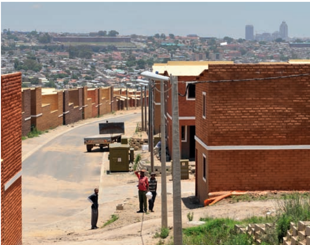
State-assisted housing with rental rooms against the backdrop of the Johannesburg skyline.
