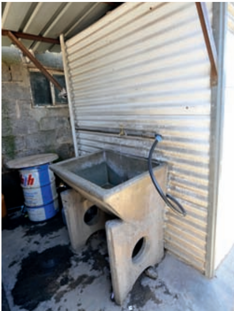
Shared washing facilities in the yard.
