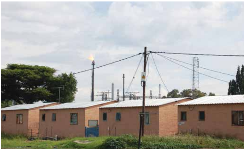
Figure 8: RDP housing in Zamdela, Sasolburg, Free State
