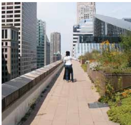
Chicago City Hall Green Roof, USA © Flickr/TouringCyclist
