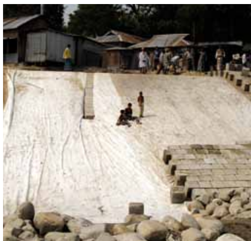
Reinforced river embankment along the Brahmaputra River in Dhaka, Bangladesh © Leila Mead/IISD
