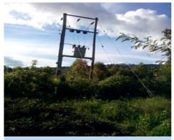
Installation of 50KVA Transformer in Rushaki ward
