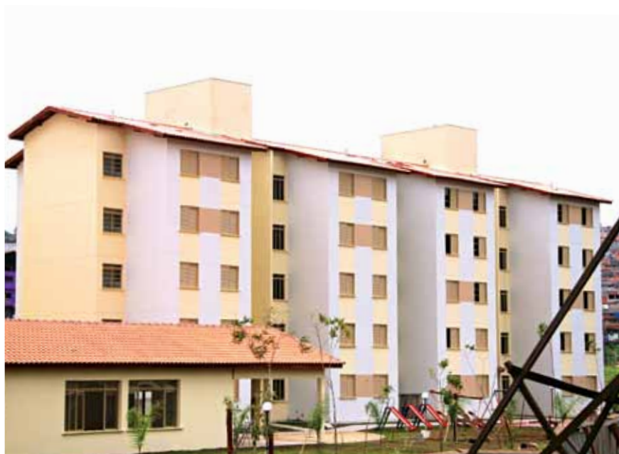
Jardim Silvina Housing Project.
