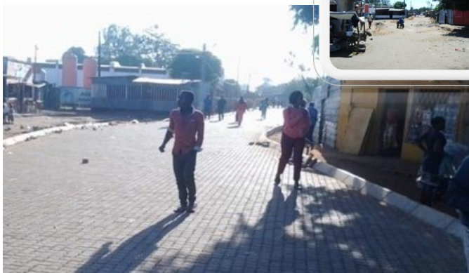
Road Construction in Chamanculo C
