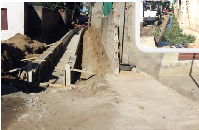
Drainage Construction in Chamanculo C
