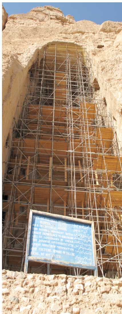
Consolidation work on the Great Buddha's niche in the valley of Bamiyan (Afghanistan)
