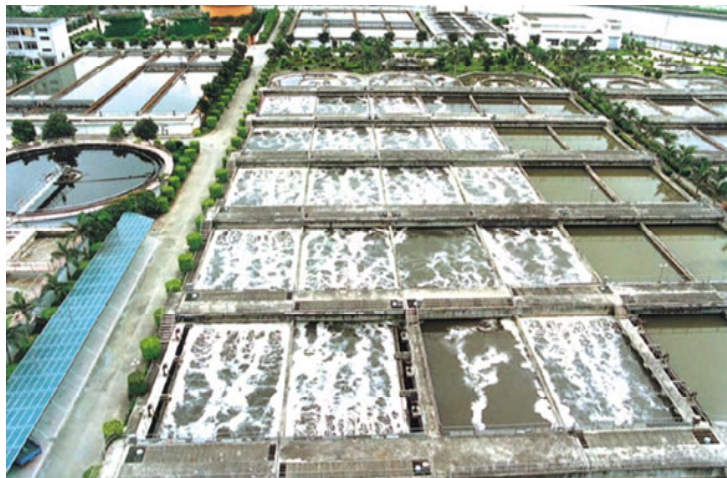
Figure 7. Shenzhen Water Treatment Plant
