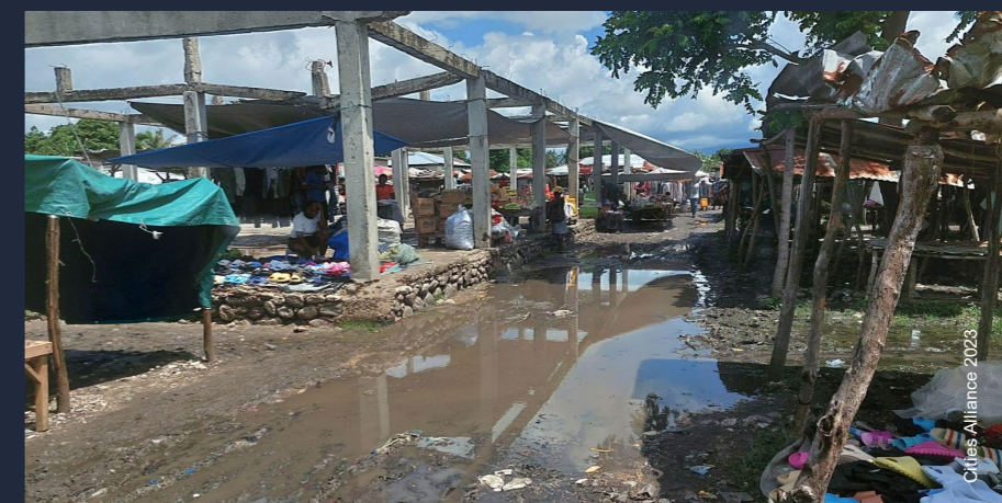
Figure 30 - Flooding of market after rainfall
