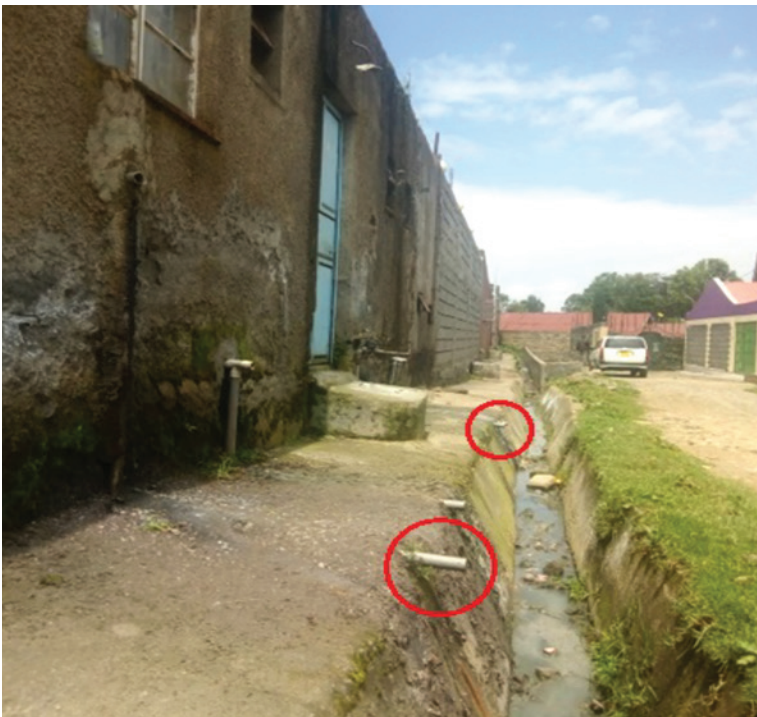
Outlet discharge of grey water into open storm water drains from the residential properties
