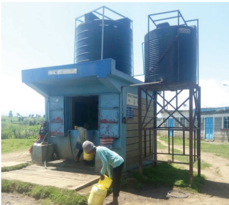
Water point (borehole and elevated plastic tanks) in residential zone 2
