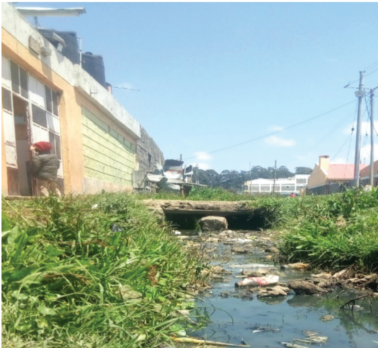
Plastics, grey water mixed with fecal waste discharged into the open drains at rear of residential buildings at the East side of zone 2
