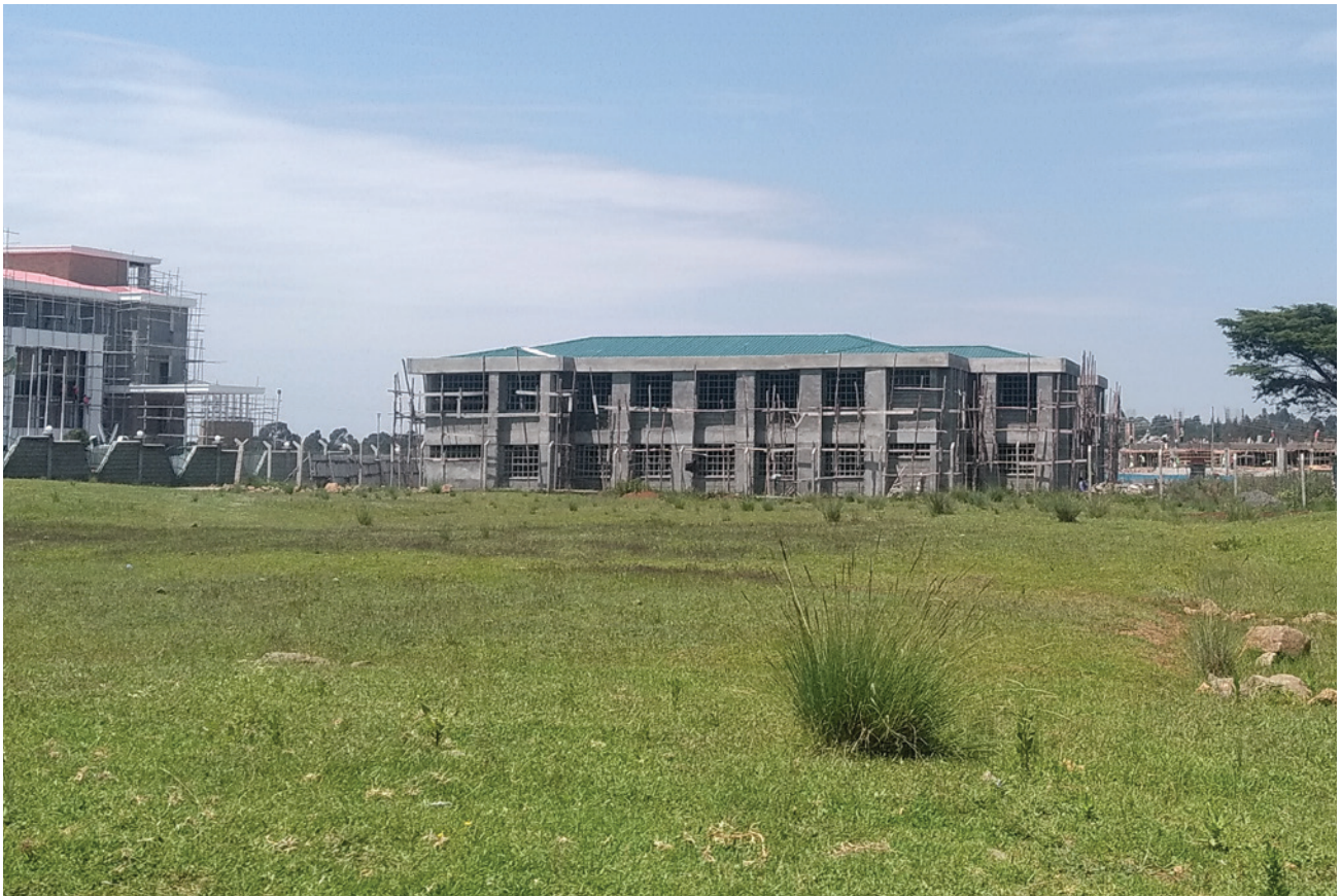
County offices under construction
