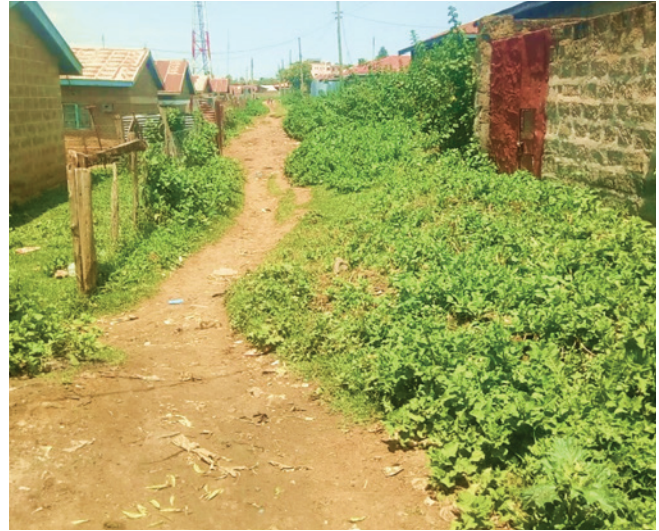
Sample of an irregular earth access road within residential zone 2
