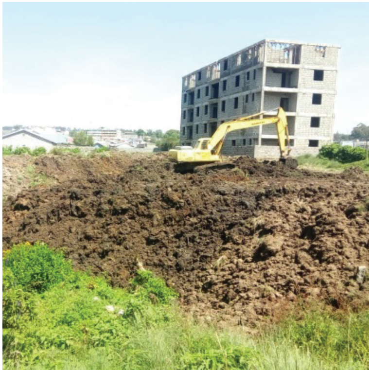
Dumping of soil excavated from a construction site on a riparian reserve
