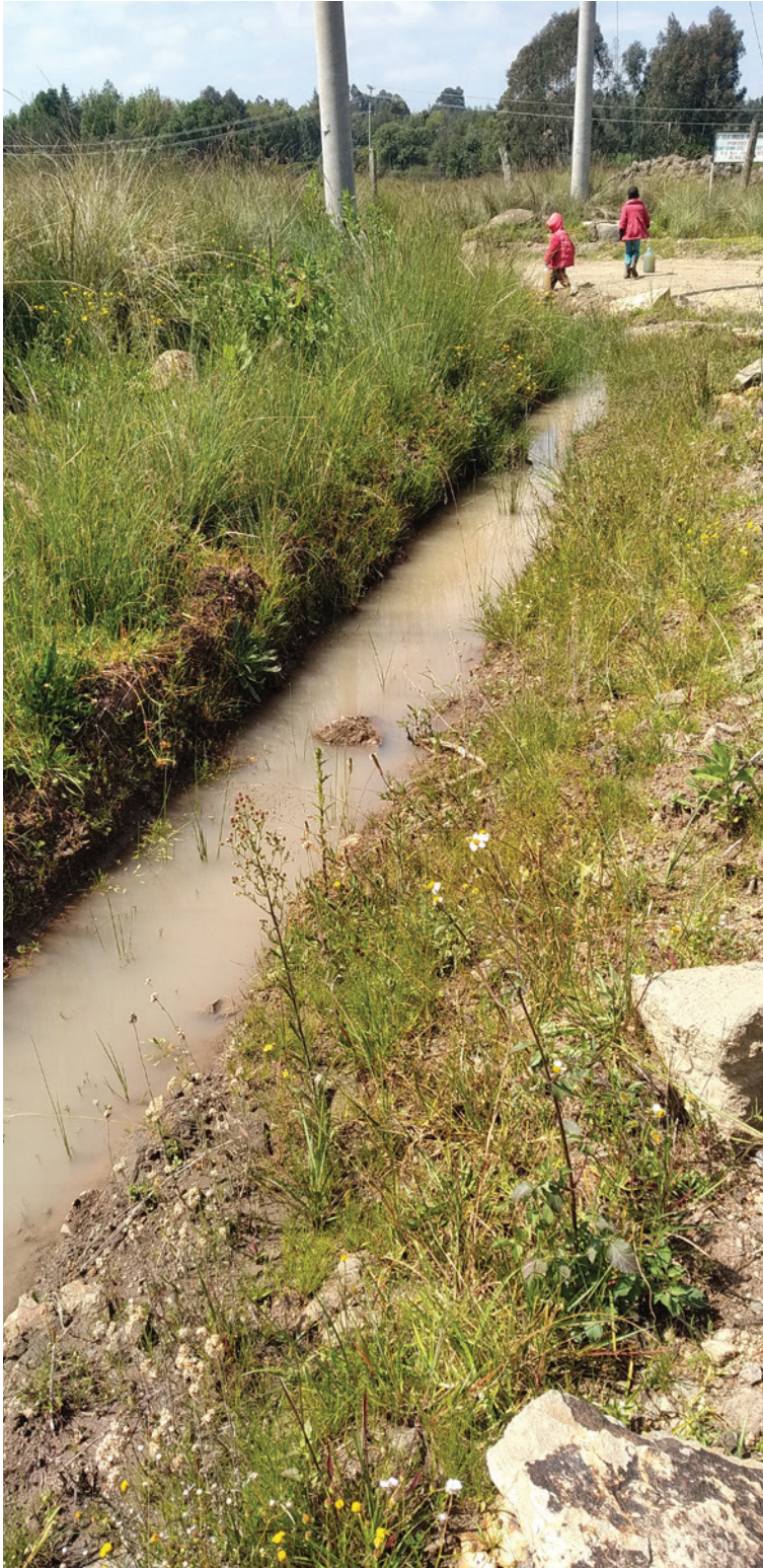
A blocked drainage systems.
