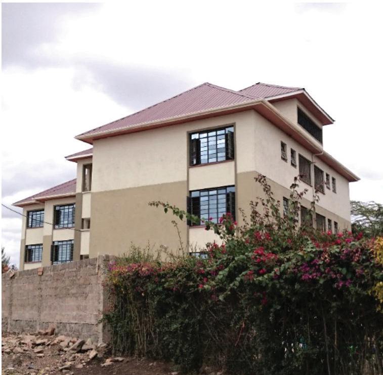
A Newly Built Apartment Block @Baraka Mwau
