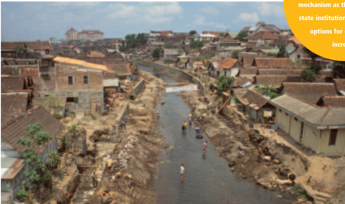
Community construction in Yogyakarta, Indonesia
