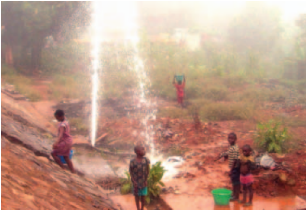
Burst water main in Mathare, Nairobi, Kenya
