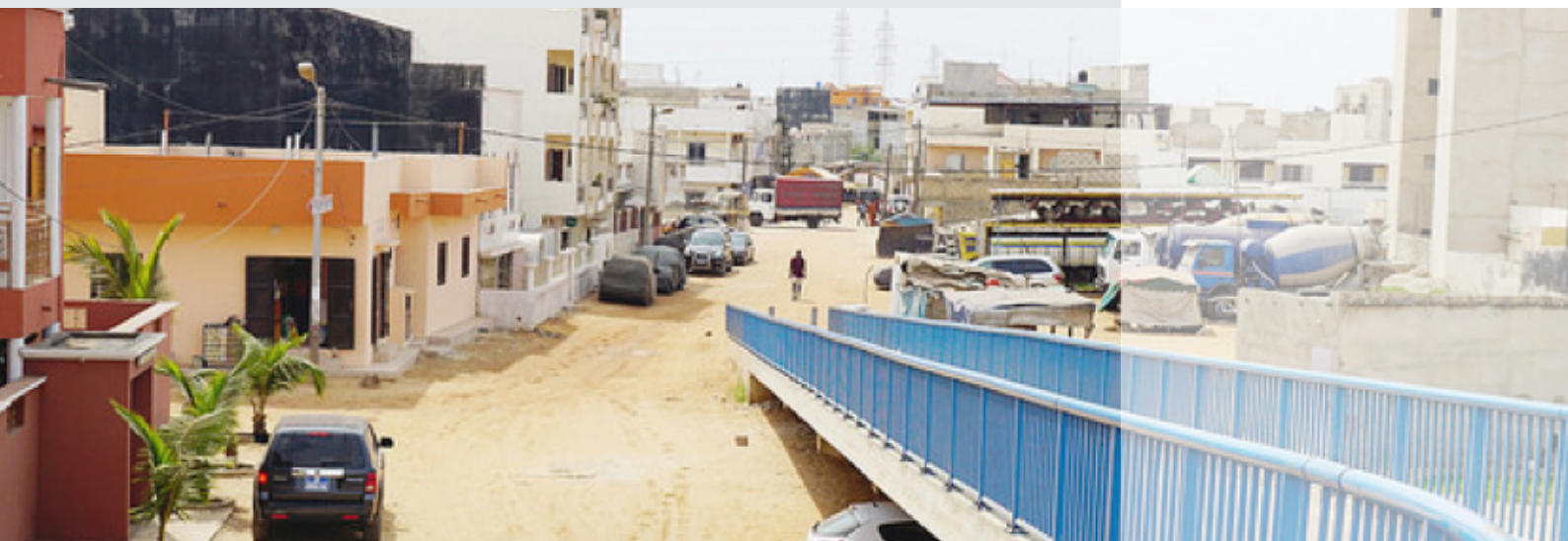
Entry point into the Municipality of Dalifort-Foirail, showing the scale of new construction and renovated houses
