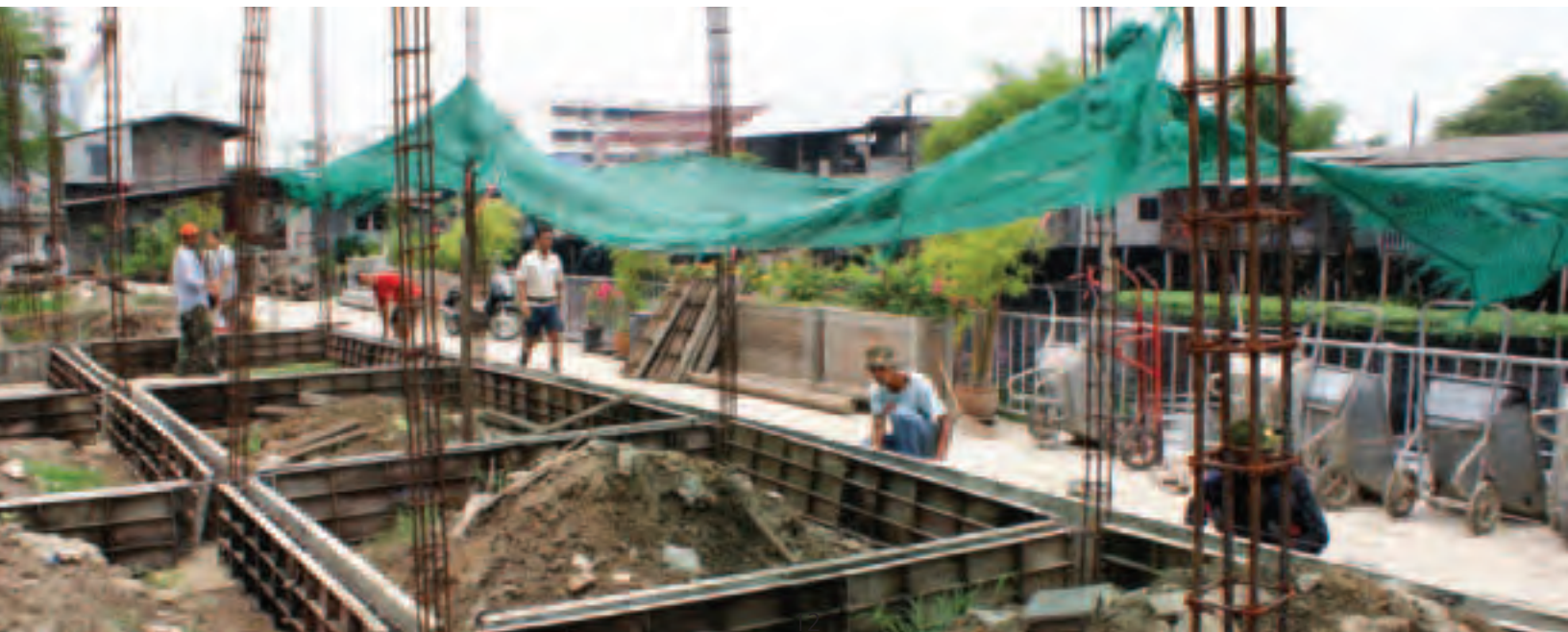
An upgrading project underway in Bangkok, Thailand. © William Cobbett/Cities Alliance
