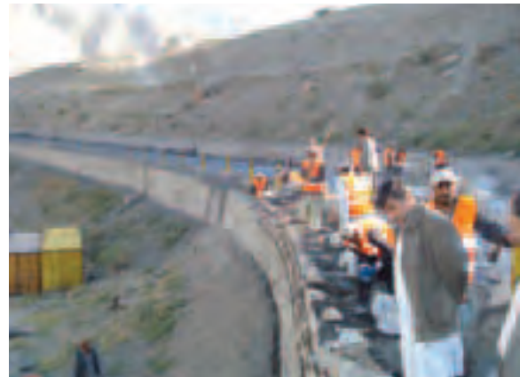
Stone walls totaling approximately 500 metres aimed to reduce the number of serious accidents was constructed on a highway in Bazarak city which is in the Panjshir province. The safety wall has already prevented numerous accidents and lives have been saved. Courtesy: USAID
