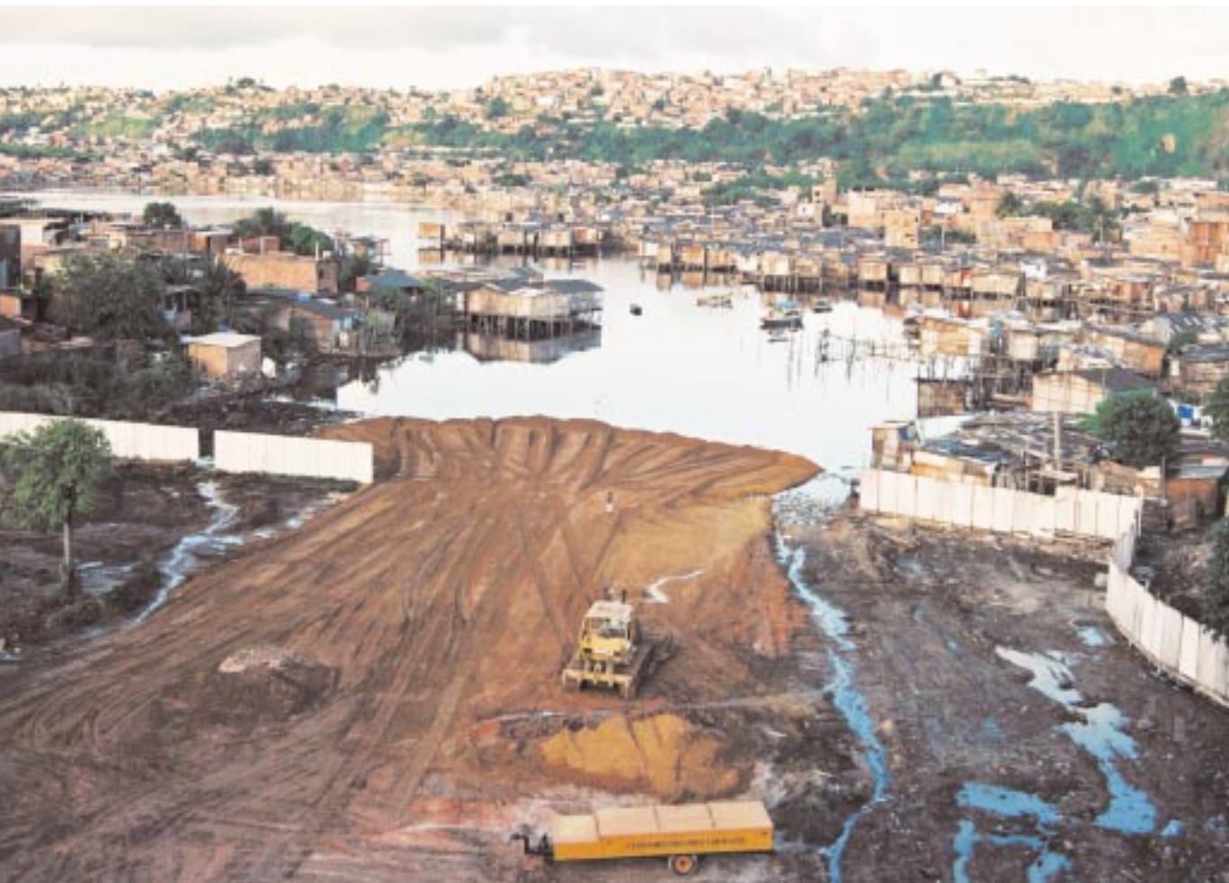
Upgrading in Salvador, Bahia, Brazil
